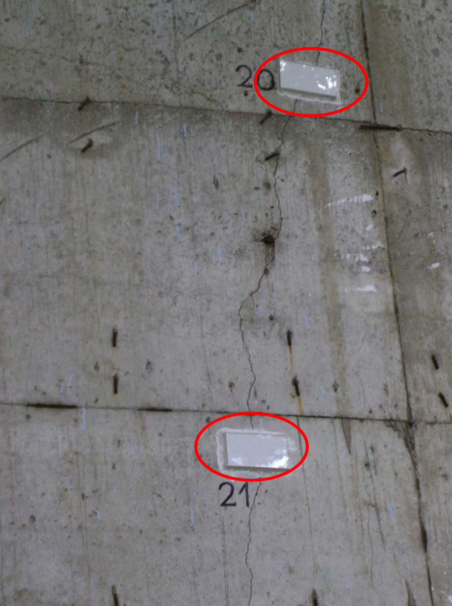
View on the glass seals glued to the cracked surface of the abutments
