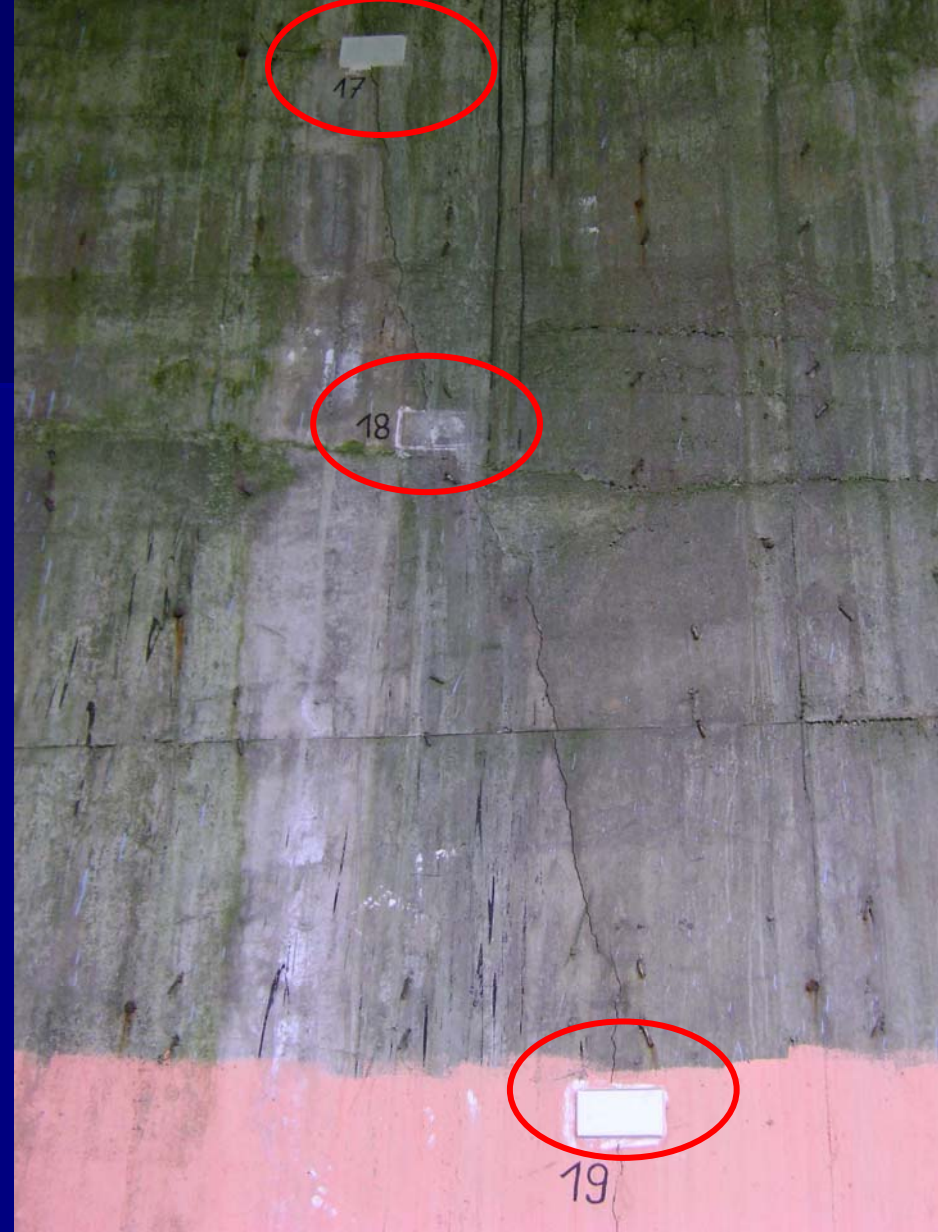
View on the glass seals glued to the cracked surface of the abutments
